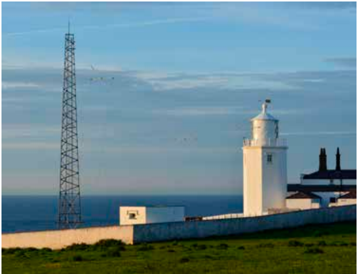
ABOVE: The same arrangement can be seen at the Lizard lighthouse, another strategic location for ship navigation. Once again, the T-wire is suspended between the top of the support mast and the lighthouse lantern.
