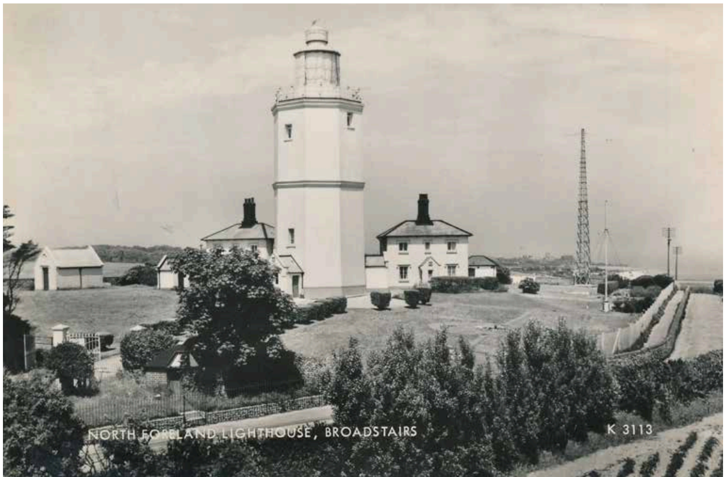
ABOVE: From a higher elevation the footpath can be clearly seen, inside the modified perimeter wall, but with the new perimeter marked out by a wire fence. Behind the lighthouse is farmland and the sea is in the distance on the right. The mast still stands.
