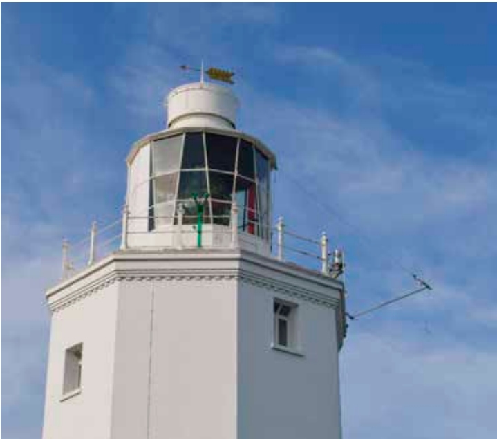
ABOVE: The three lines of the T-wire travel from the mast and are fixed to the lantern of the lighthouse.
