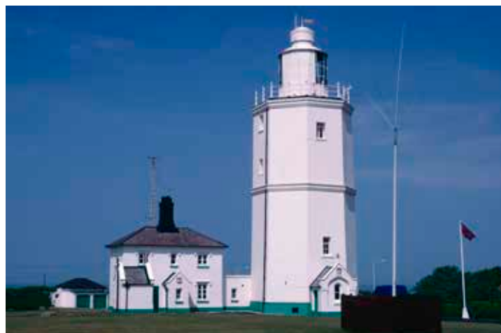
ABOVE: The antenna just to the right of the tower was to be found at South Foreland too. This was the radio beacon at both stations. Note, the wooden flagpole has been a long-time feature of the station, essentially unaltered over many decades.
