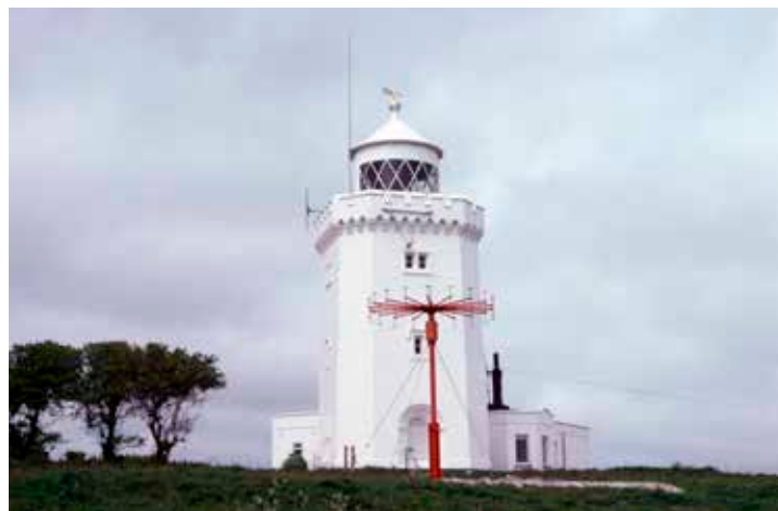
ABOVE: In the mid-1980s, there was a VHF D/F antenna for use by the Coastguard, here seen as the red apparatus at South Foreland. The same antenna is shown BELOW at North Foreland on a tall mast behind the cottage.
