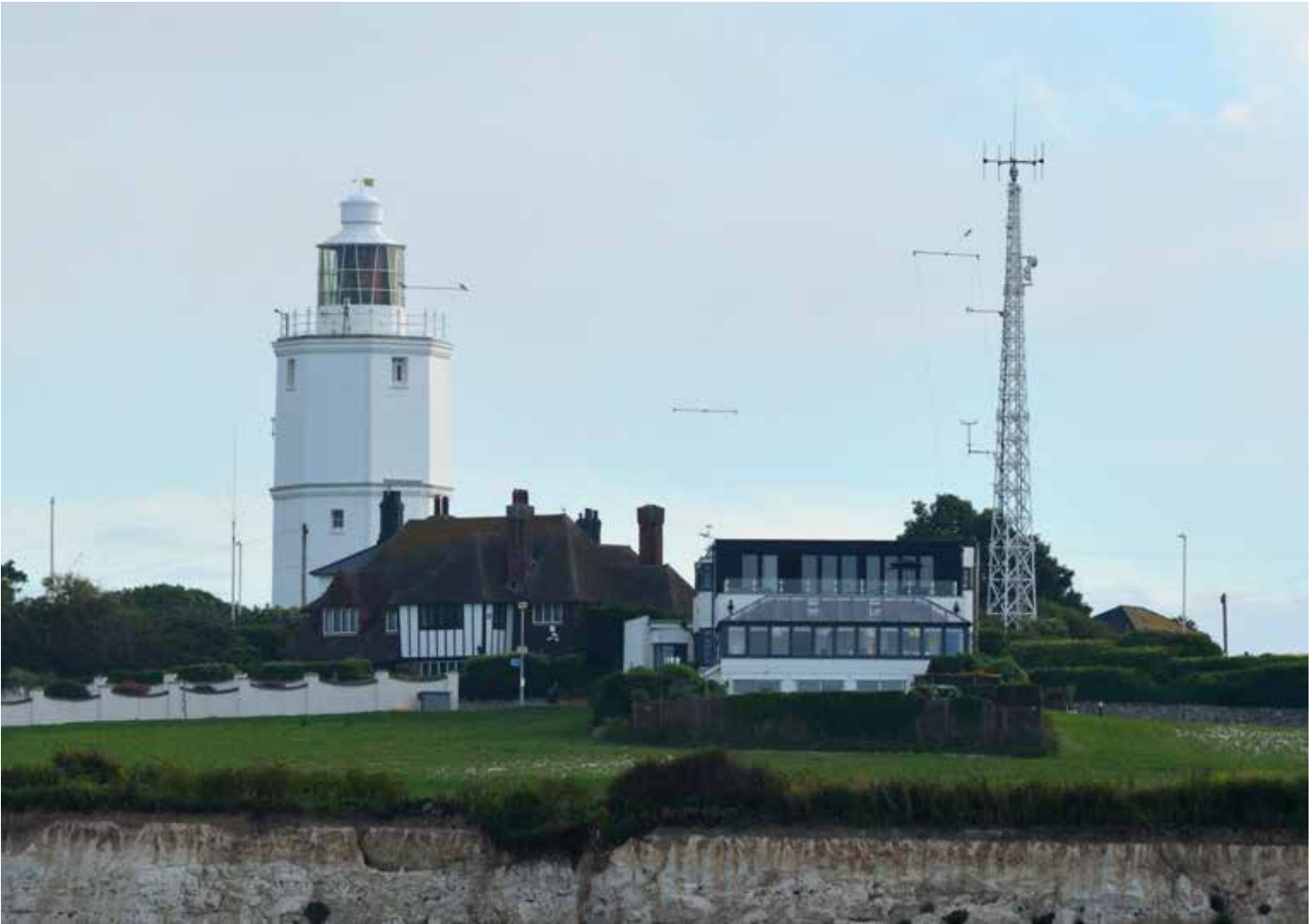
Above: In this photograph, taken from the sea in 2021, a number of antennas are visible attached to the mast and fulfill different roles. Less visible are the three lines stretched between the mast and the lighthouse, known as the T-wire antenna. (The foreshortening effect of the telephoto lens makes the private house look much closer to the lighthouse site than it is.)
