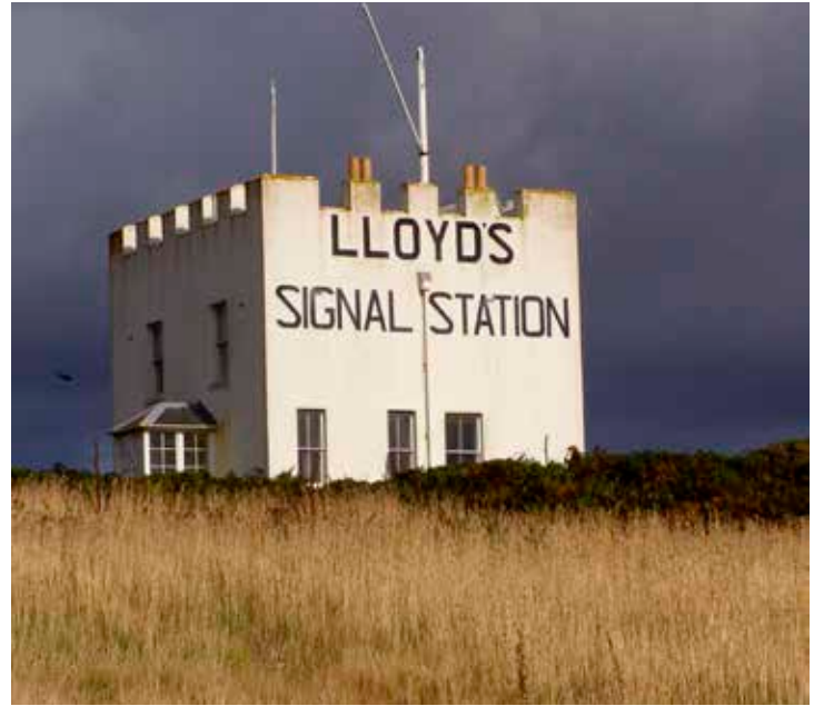
ABOVE: The Lloyd's Signal Station at Bass Point on the Lizard, Cornwall UK. The whitewashed two-storey masonry building has a five-sided full-height bay on its south wall, and a flat roof surrounded by a castellated parapet. It is 9.1m high and has a lookout structure with a stout mast for flag signals on its roof.
